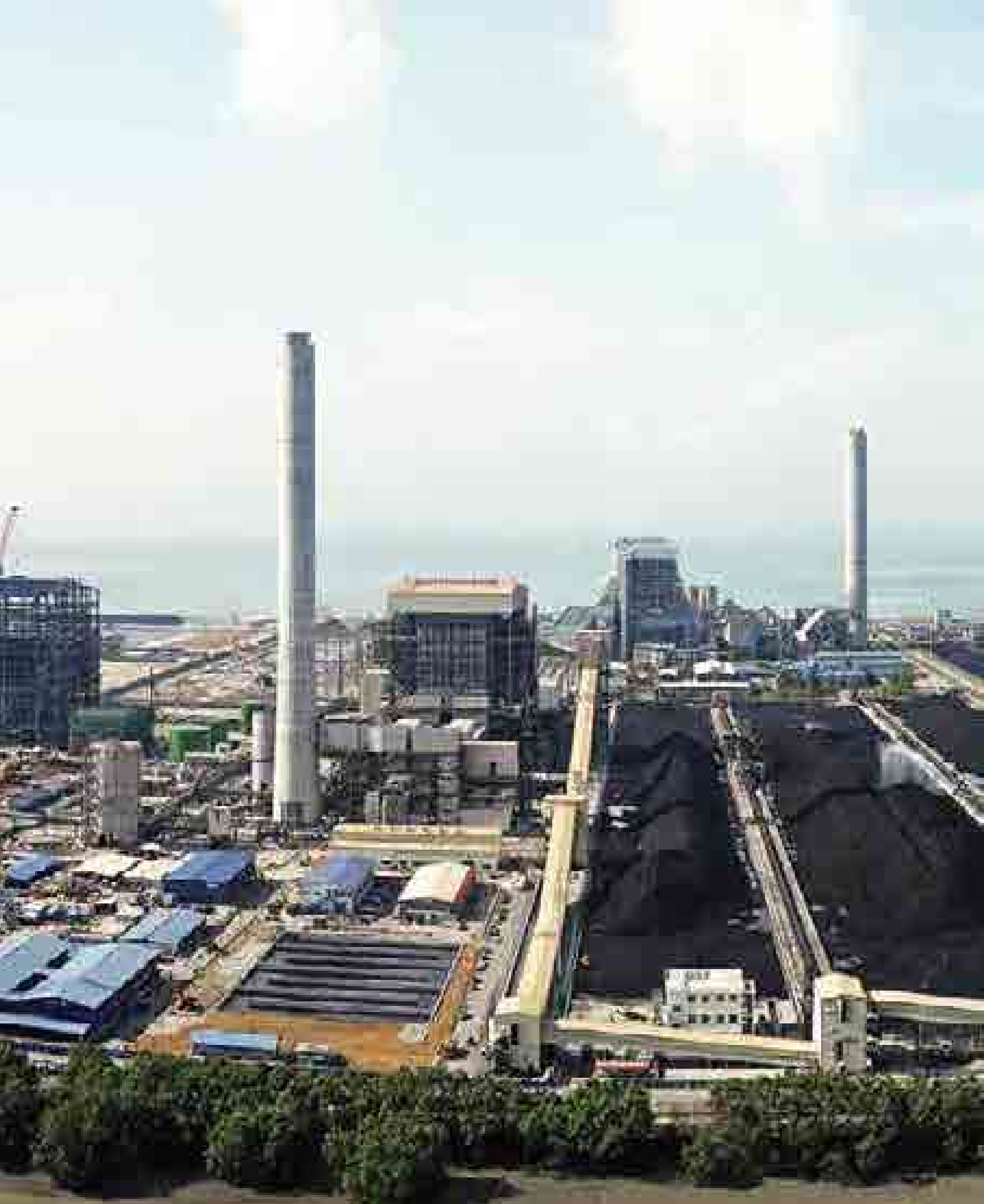
Manjung Unit IV (1x1,010MW) Coal-Fired Power Plant, Manjung, PERAK
