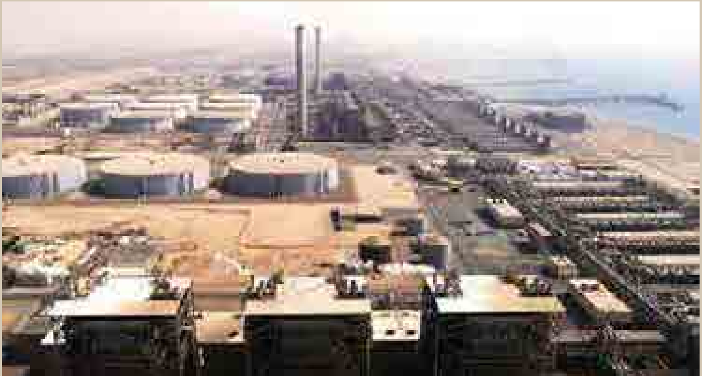
TNB REMACO has been operating the Shuaiba power and distillation plant owned by Kuwait's Ministry of Electricity & Water since 2013
