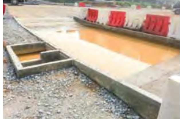
Wheel washing facility provided at site entrance
