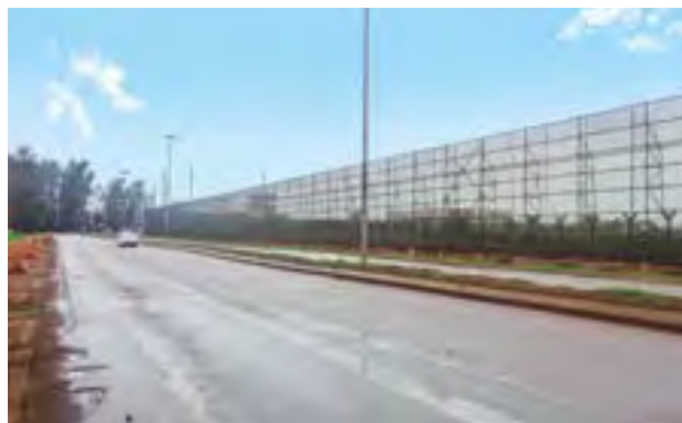
Airborne dust mitigation panels at Kuantan Port
