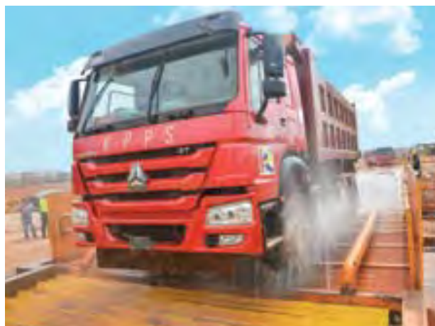
Wheel washing facility to minimise dust pollution
