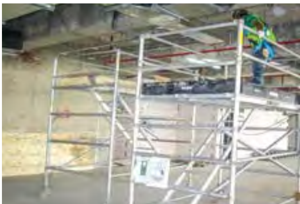
Working platform erected for workers at site
