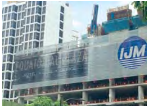
Installation of screen system at construction site
